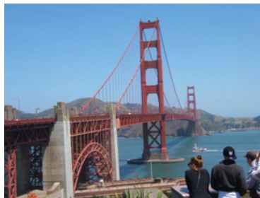
Viewing the Golden Gate Bridge
